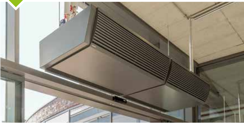
Tandem 300 Door air curtains with Tandem technology. Ambient air and heated air stream for effective cold air screening.
